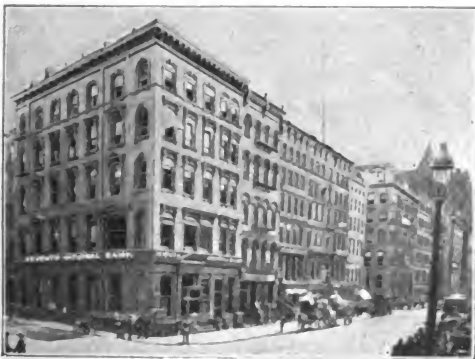
SEVENTH NATIONAL BANK, BROADWAY AND JOHN STREET.
